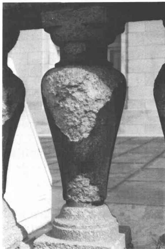
Fig. 7. Photograph of salt damage to one of the marble balusters in the balustrade of the patio and west side of the Pan American Union Building, Washington, D.C. The black area is an outer layer composed mostly of gypsum mixed with soot. The white area is composed mostly of gypsum.
