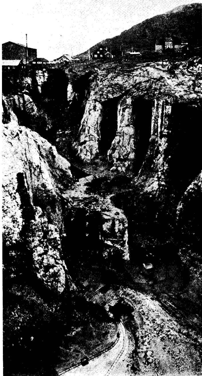
Fig. 1. View of Ivigtut Cryolite Quarry, looking east (autumn 1937). In the left foreground, the foot of the elevator pillar, and, to the right of this, the entrance to the lower tunnel flanked by the area from cote —55 to —60. Above the excavator to the right, the western part of the eastern quarry.
